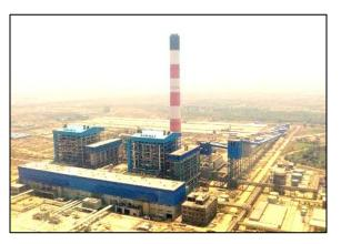
L&T-Sargent & Lundy (L&T-S&L) was responsible for Complete Basic and Detail engineering services of STG Island including its auxiliaries. The project was executed through package route for Boilers and BOP. L&T-S&L extended full engineering support for plant integration activities and also provided necessary site support.
