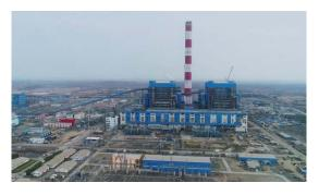
With steam parameters of  $600~^{0}$ C and  $270~\text{kg/cm}^{2}$  pressure, these units have been designed to consume less coal and produce the equivalent of power in comparison to supercritical plants; L&T-MHPS supplied the boilers and steam turbine generators.
